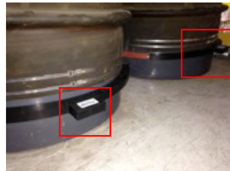
Fig. 6 The installation of bushing type PD sensor
