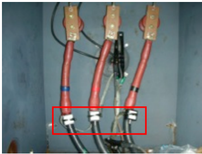
Fig. 8 Installation of UHF PD sensors
