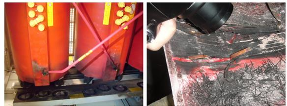
Fig. 2 Insulation breakdown initiated by heat aging (poor connection)
