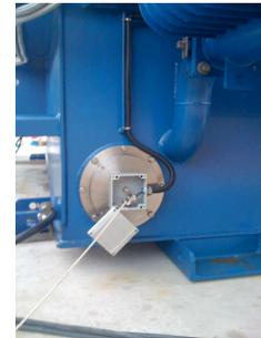
Fig. 5 Hatch type of UHF sensor
